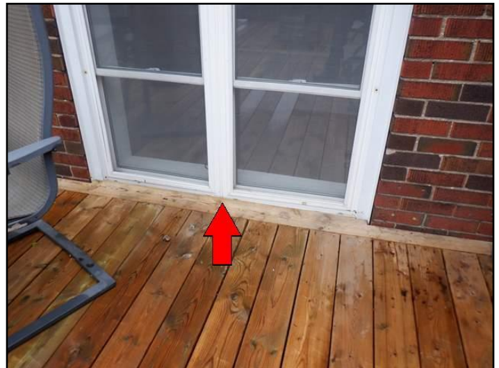
Window sill below deck surface
