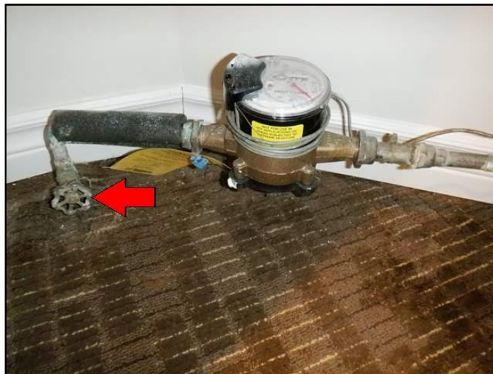
Front of the basement
